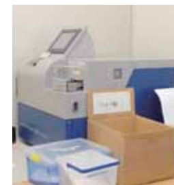
The explosive detection equipment is installed in the office and we provide thorough security for export cargo.
